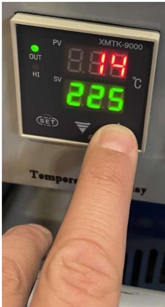
Photograph 3: The temperature is raised with an up arrow.
